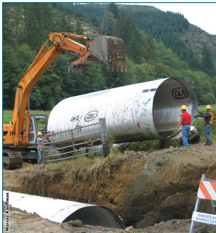
Crews work on a stream restoration project
